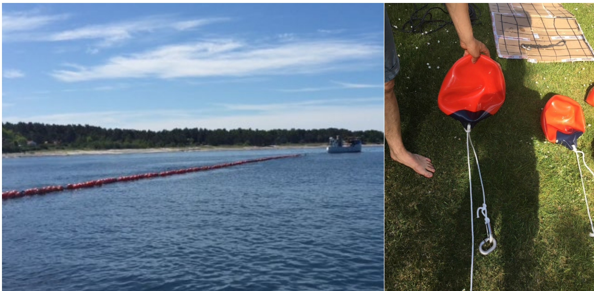
Figure 7. Left: A net with floats towed after the work boat. Right: Quick-links to buckle the nets were prepared on the anchor lines. A float at each quick-link keeps the anchor line afloat while waiting for the nets to be towed in position before fastening.
