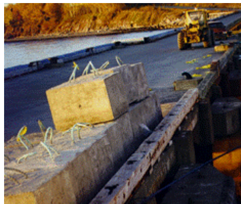
Figure 32 Anchor blocks loaded on dock
