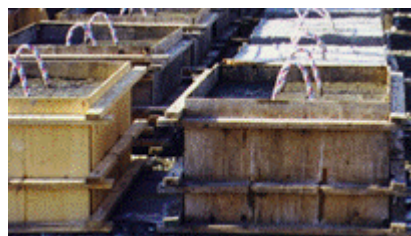
Figure 5 Square concrete block anchor
