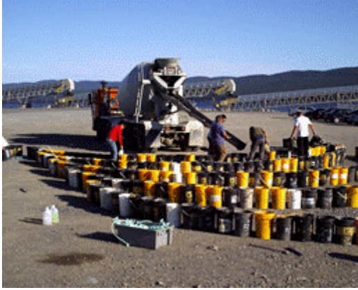
Figure 17 Production of compensation ballast weights
