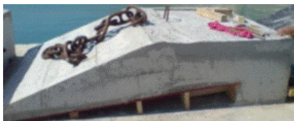
Figure 4 Wedge-shaped concrete block anchor
