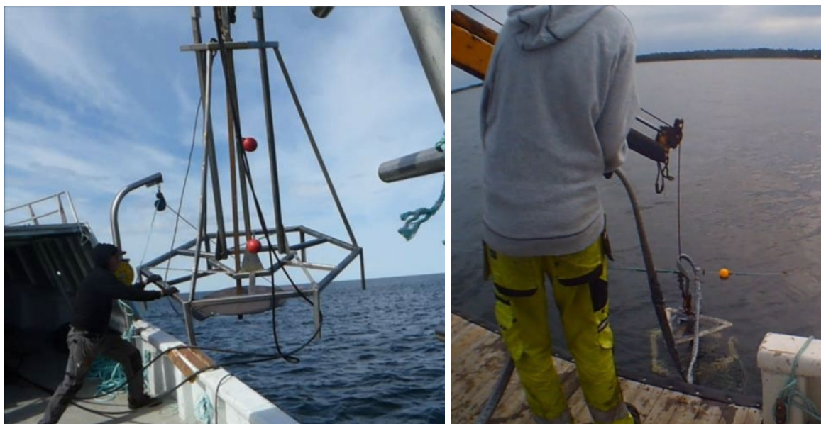
Figure 5. Left: Setting of the 20 helix side-anchors in 2016. It was hard to maneuver the swinging drill-rig from a classic round-bottomed fishing boat. The original big plates shown in the picture were soon exchanged to smaller plates that could penetrate the sand-bottom. Right: Setting of 27 vertical anchors in 2017. This job was done with part of the rail removed, a new wooden deck, and perfect weather conditions.
